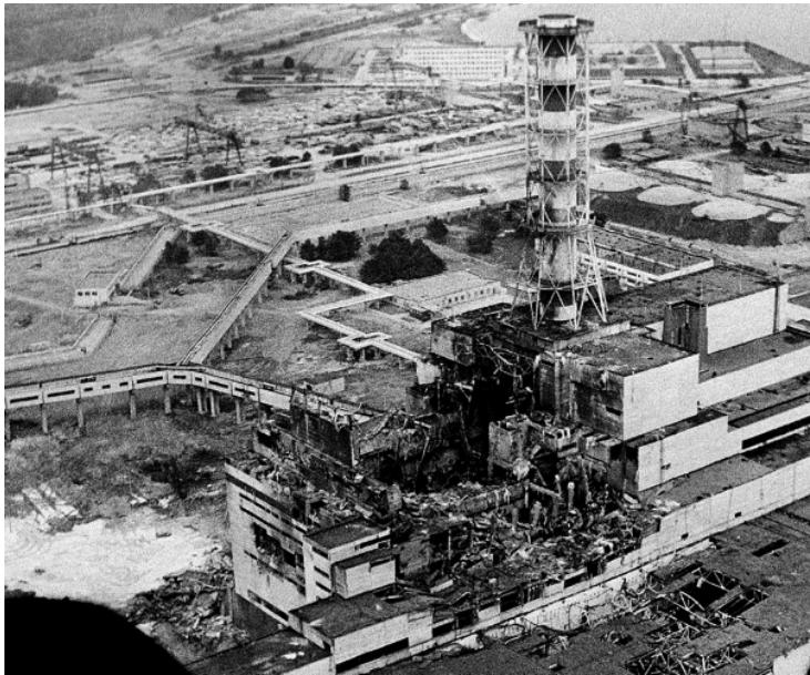
View of the reactor No 4 after explosion
